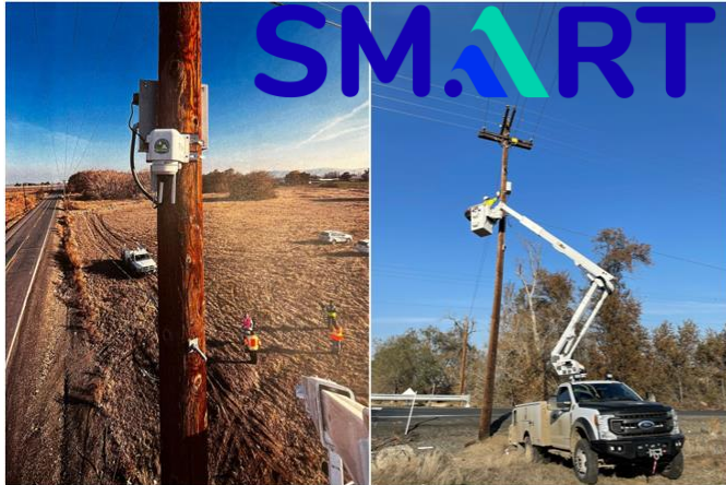
Edge AI Device for Traffic & Road Conditions Monitoring and Hazardous Events Detection
